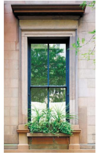
A two-over-two, double-hung window with full window enframent with incised detailing.
