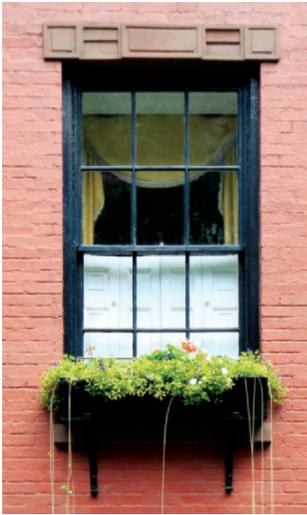
A six-over-six, double-hung window with brownstone lintel and sill.
