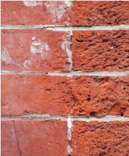
The negative effects of abrasive cleaning or sand blasting on brick (shown on right).
