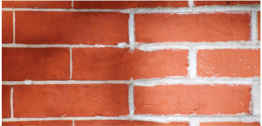
In a good repointing job (left), the new mortar matches the existing mortar in color, hardness, and joint profile. A poor repointing job (right) can destroy the original appearance of the building. Here, the mortar joints are too wide and the composition of the mortar is too hard.
