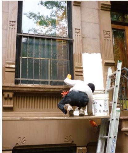
Paint being removed from a brownstone facade with a proprietary chemical peel.
