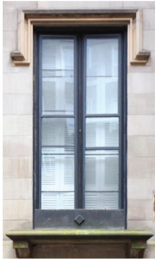
A multi-paned casement window with a molded eared stone lintel and bracketed sill.
