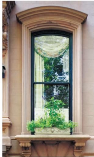
A segmental-headed, one-over-one, double-hung window with a bracketed stone lintel and molded enframent.
