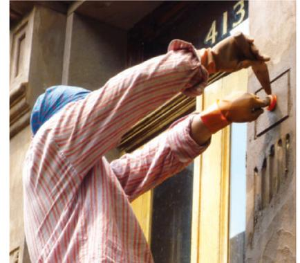
A brownstone facade being partially resurfaced with matching stucco.
