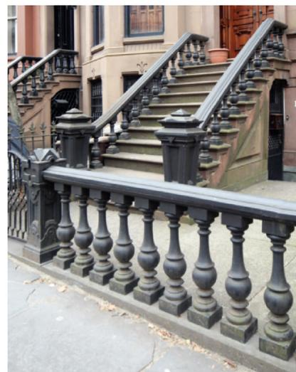
Cast-iron areaway fence and stoop rails on a neo-Grec style rowhouse.
